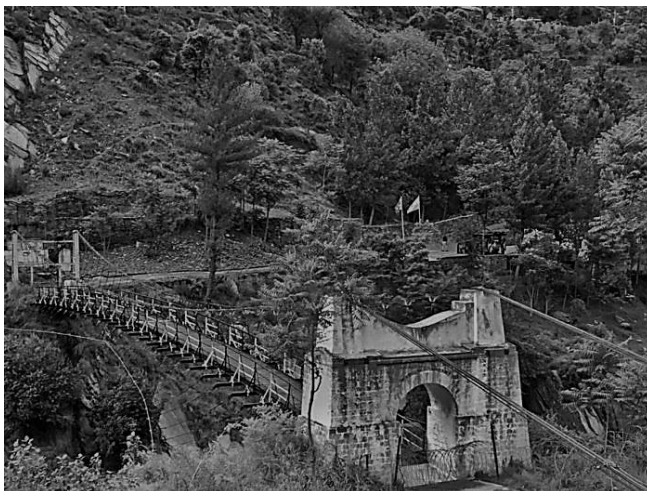
Tithwal crossing bridge over Kishan Ganga River, Source: Kashmir Radio Chinar
